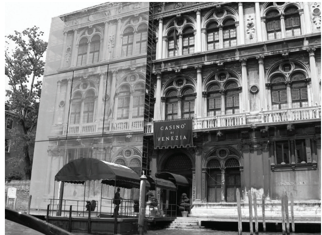
Figure 1: Photo of the Casino di Venezia in Venice, Italy undergoing renovations behind scaffolding wrapped in an image of the building. 8
